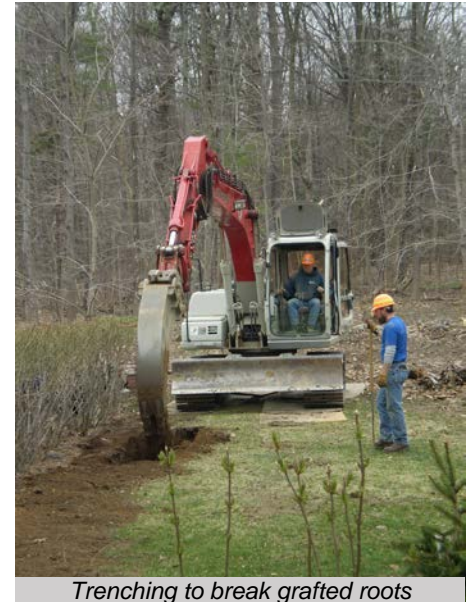
Trenching to break grafted roots
